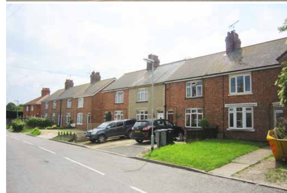
Fig 171 and 172: Red brick terraced properties located towards the junction with the A15 form one of the most uniform and coherent residential groupings within Character Area 8
