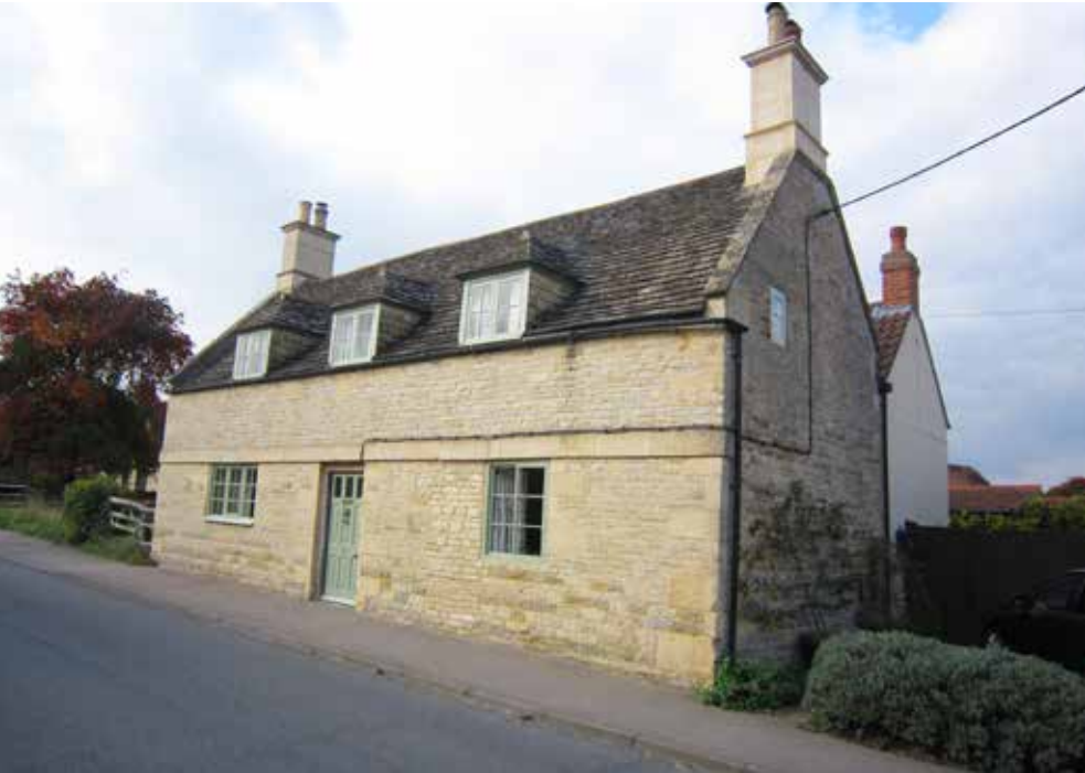
Fig 56: Bindon House, dating from 1760, is one of several characterful historic properties to be found within Character Area 2
