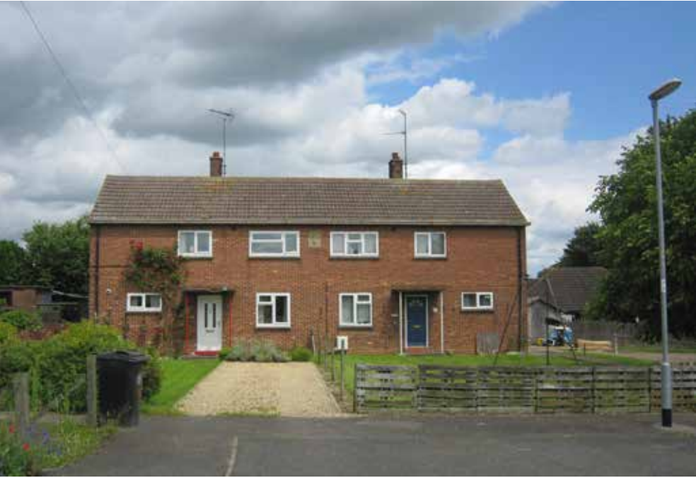
Fig 82: Buildings throughout Maple Avenue share the a common materials palette architectural language
