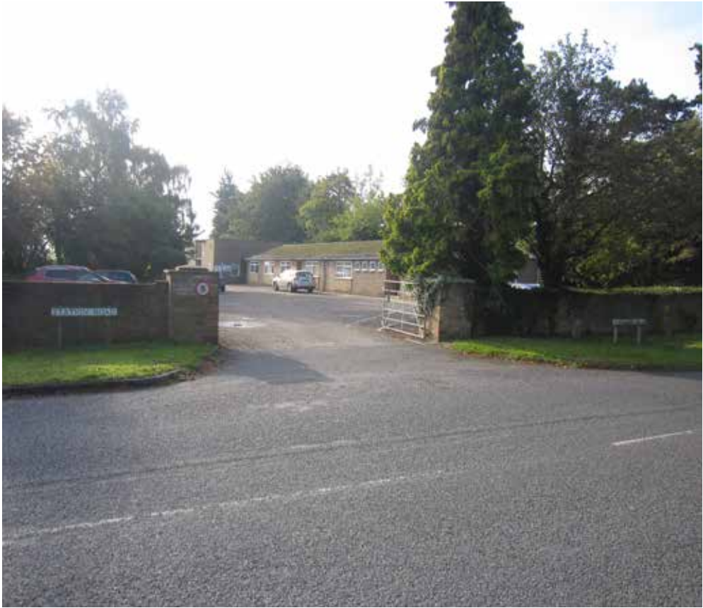
Fig 135: LCC Highways Depot lies set back from Station Road, and is generally well-screened in views from the roadside by boundary walls and planting.
