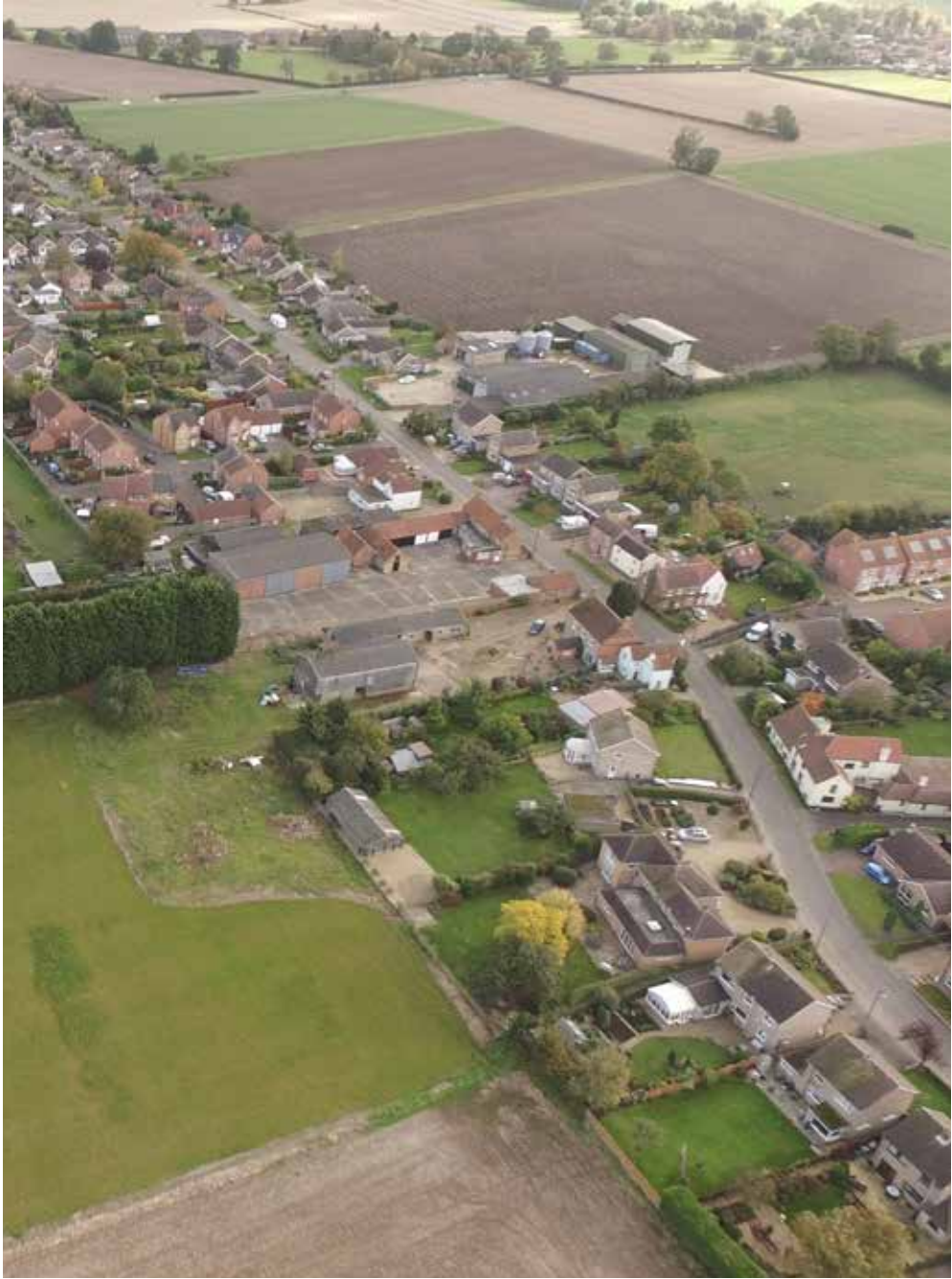
Fig 50: Regular plot arrangements and building positioning give way to more ad-hoc and varied historic layouts as Northorpe moves away from the A15 towards Northorpe Lane
