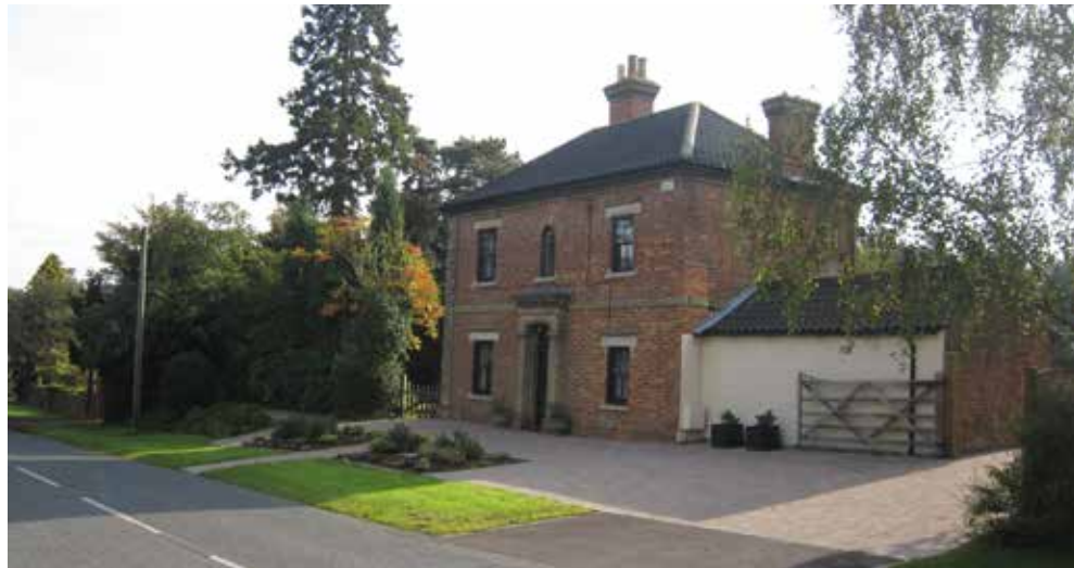
Fig 143: No. 1 Swallow Hill is one of the stand-out dwellings found along Swallow Hill, with a simple yet elegant form topped by a hipped roof punctured by towering red brick chimney stacks
