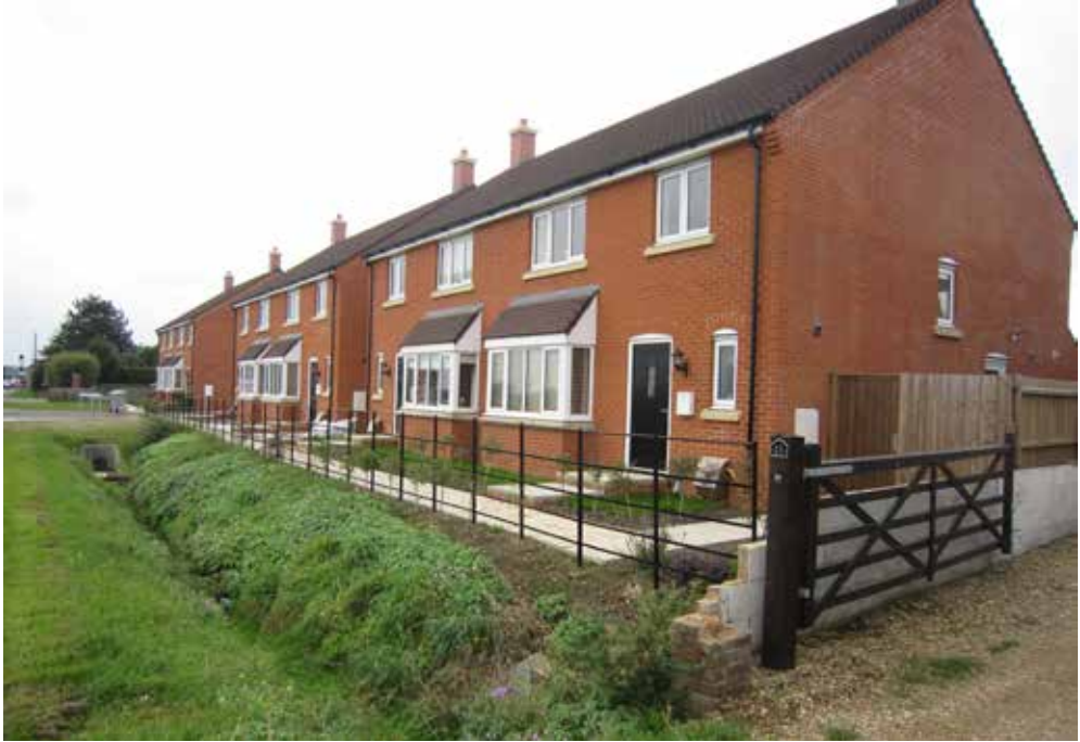
Fig 51: At the junction of Northorpe and the A15 is a row of semi-detached dwellings that present a strong frontage on to the trunk road
