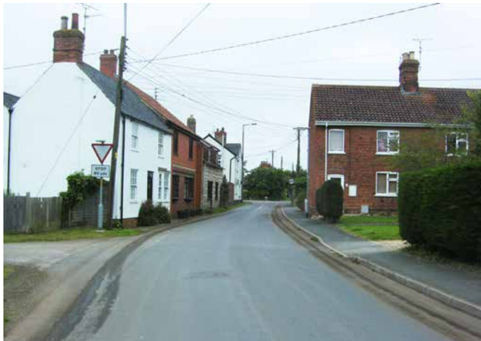
Fig 195: Terraced buildings on the southern side of Church Street where it meets with the A15 are positioned right on the road, creating a well-defined edge to this side of the street and a strong sense of enclosure
