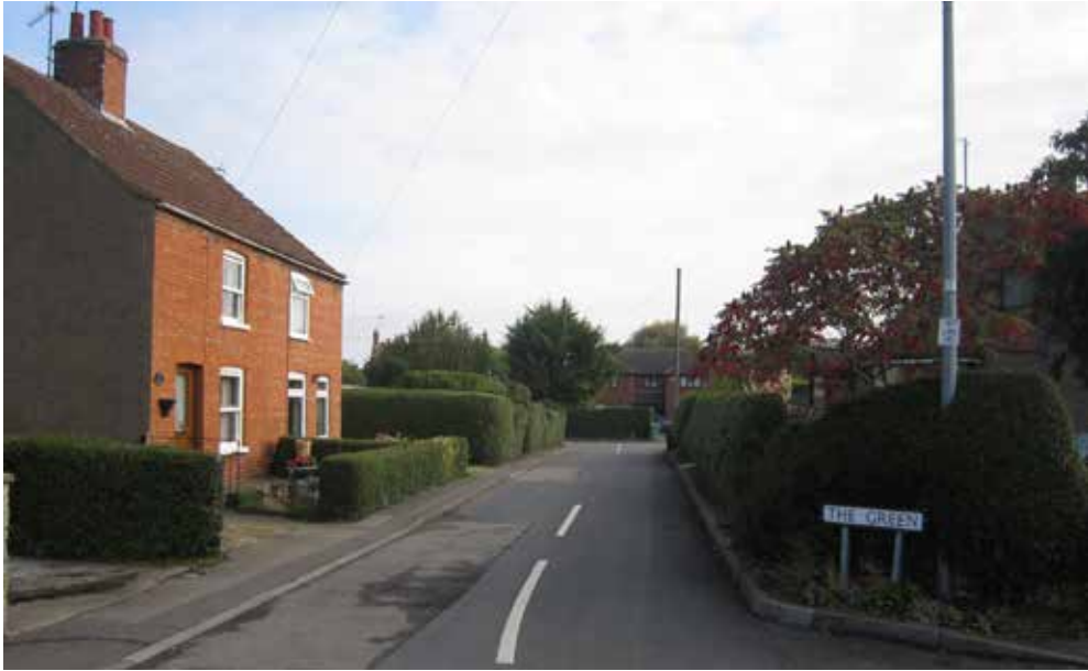
Fig 109: Older routes such as The Green that links through to Crown Lane has relatively narrower profile, and are often edged by buildings that are positioned close to the roadside, creating a more intimate street
