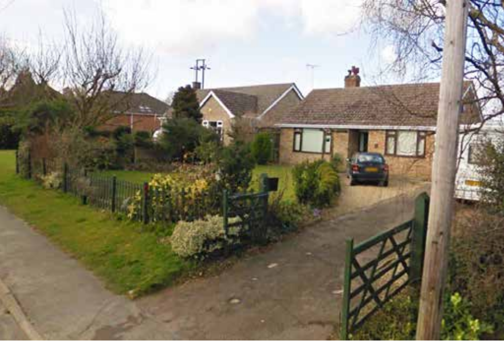
Fig 141: Single-storey residences finished in various tones of brick occupy the northern side of Swallow Hill just before it meets Station Road
