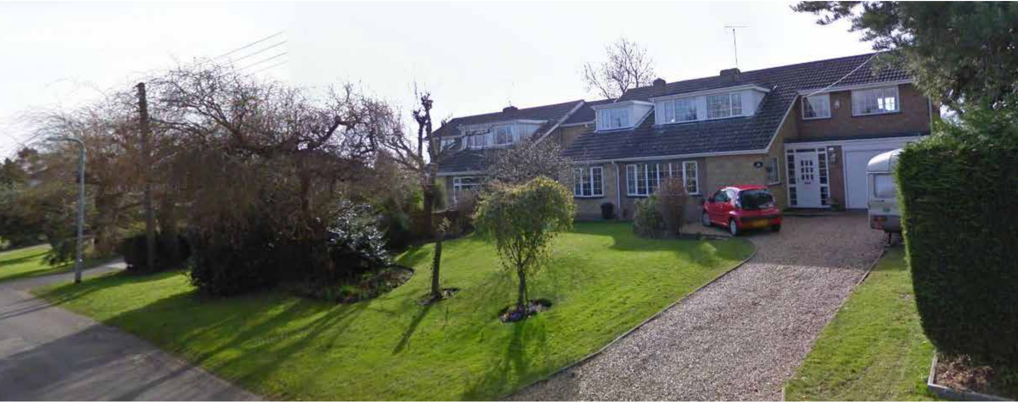
Fig 156: One and a half storey dwellings of 1970's construction with later extensions, represent one of the dominant dwelling types found along the western edge of Obthorpe Lane
