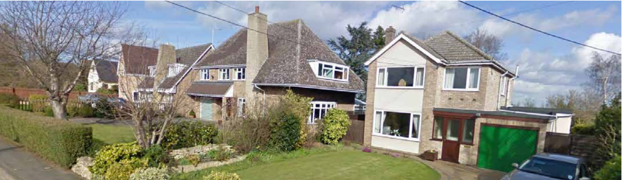
Fig 152: Though buildings differ in scale and appearance, they are all positioned along a similar building line behind generously sized front gardens
